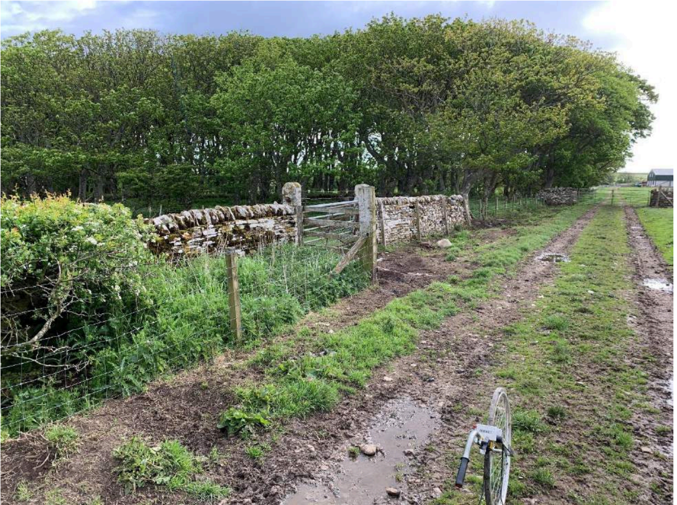
4770 - End of the hedge to the eastern end, showing gap within fenced area, field gate and section of wall before woodland edge
