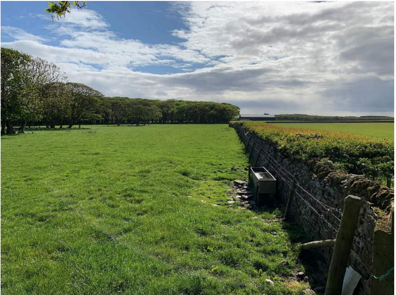
4784 - View of the north side of the boundary wall that runs parallel with the hedge
